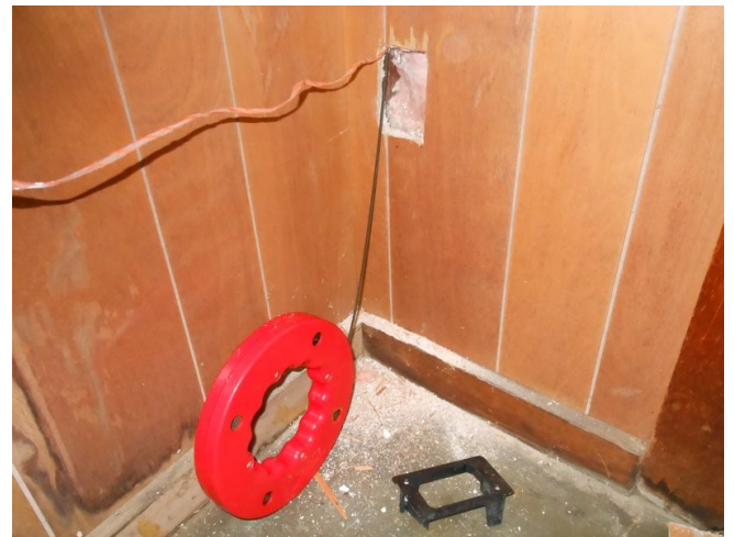
Feeding nylon string, and a wire up from the bottom of the wall to the ceiling. This is where the single sensor will be.
