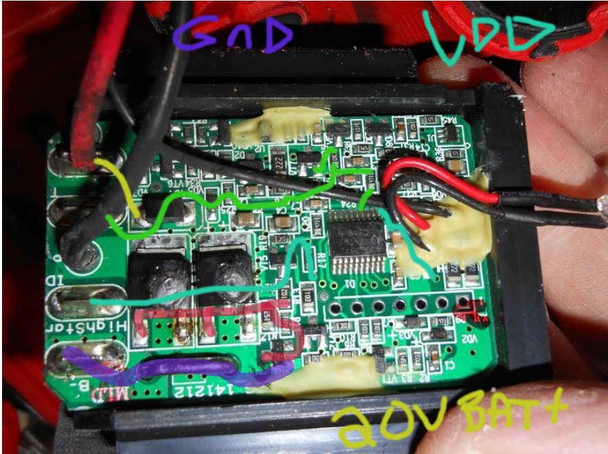
Figure 3: Rough signal path for board. When switch is pressed, there is 20V on the tab of FET. I believe the FET must've overheated and shorted (perhaps counterfeit, or just not spec'd right). Though Right pin is to GND. Maybe it's a current limiter, not a FET, allowing Tab when V+ to be dropped down and current will flow. Too bad I wasn't able to stop using the drill before both FETs failed. I could've read one of them for a part #.
