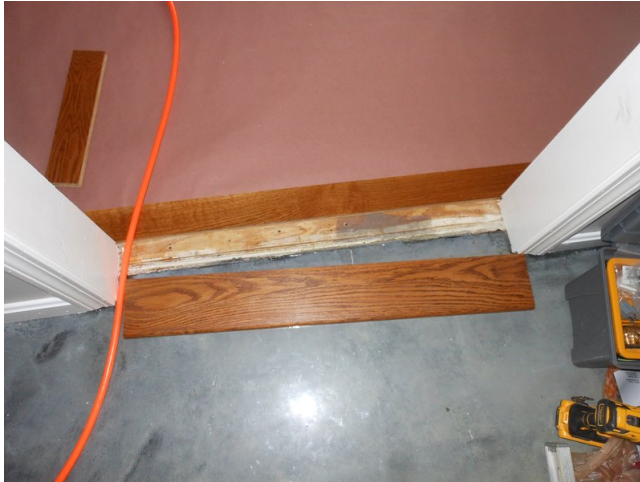
Figure 8: This transition piece between rooms was custom made.
