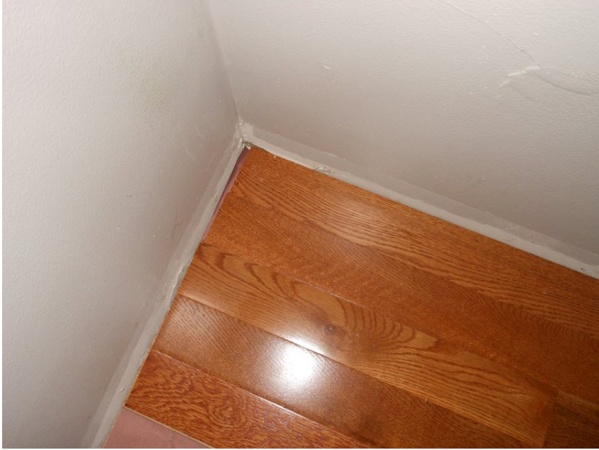
Figure 9: Some spacew was left on the east and west sides of the wall.
