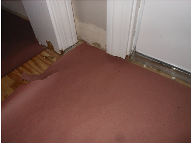
Figure 2: Rosin paper stapled to plywood. On the left is the closet, and that gap was later filled in.
