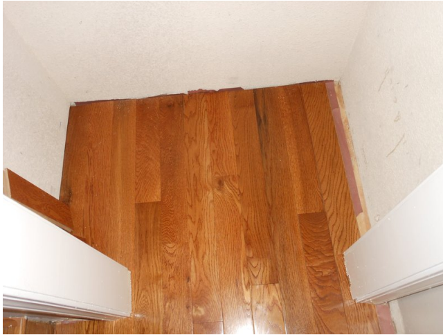
Figure 12: Pieces that weren't as good are put in the corners, and in the closet. Higher grade hardwood has less poor or off-colour pieces.
