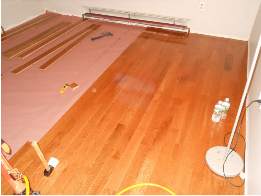
Figure 10: Progression of the wall is generally one line at a time.
