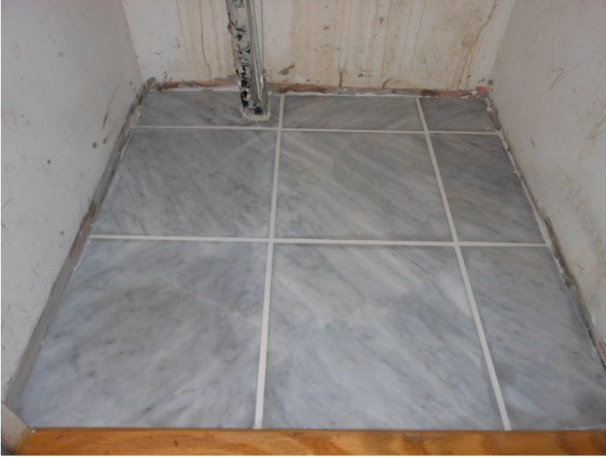
Figure 4: Grout in place. Now need to add trim. The grain was tried to be placed in a harmonious pattern., although the back pieces were not 100% perfect. The first impression from others was that the grout lines were too big. This may be true, but it looks good even when bending the tradition of small grout lines for marble.
