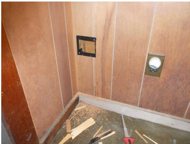
*Low profile two gang wall plate installed.*
