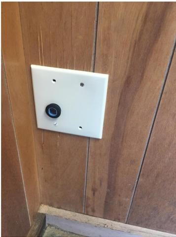
Here's how the outlet looks just before putting the final machine screws in. It was important to buy a "non breakable" wall plate (essentially a bendable more rubberized one), as the normal wall plate, simply shattered when drilled into. The non breakable version worked well with the drill.
