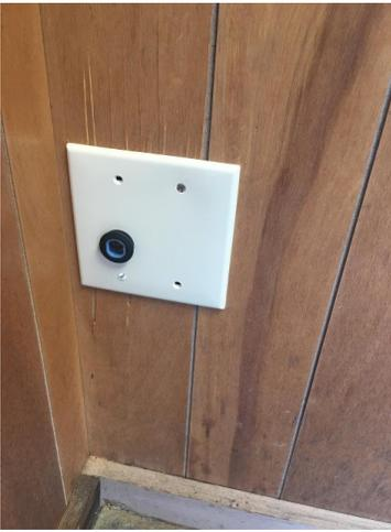
*Here's how the outlet looks just before putting the final machine screws in. It was important to buy a "non breakable" wall plate (essentially a bendable more rubberized one), as the normal wall plate, simple shattered when drilled into. The non breakable version worked well with the drill.*
