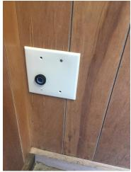
Here's how the outlet looks just before putting the final machine screws in. It was important to buy a "non breakable" wall plate (essentially a bendable more rubberized one), as the normal wall plate, simply shattered when drilled into. The non breakable version worked well with the drill.
