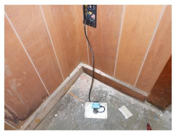
Installing the single sensor. I used ethernet as the power line. I also used a passive PoE adapter on both sides to transfer the power onto the ethernet, and back out to a 5.5, 2.1mm barrel plug
