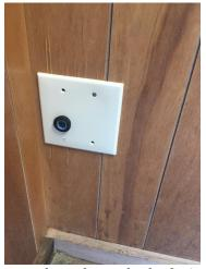
Here's how the outlet looks just before putting the final machine screws in. It was important to buy a "non breakable" wall plate (essentially a bendable more rubberized one), as the normal wall plate, simple shattered when drilled into. The non breakable version worked well with the drill.
