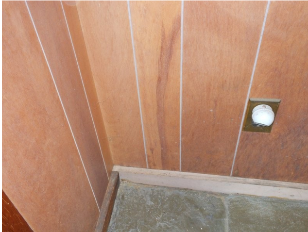
Choosing location for the sensors. Keep in mind, that the laser diode path must remain open. This is where the main board and sensor will be.
