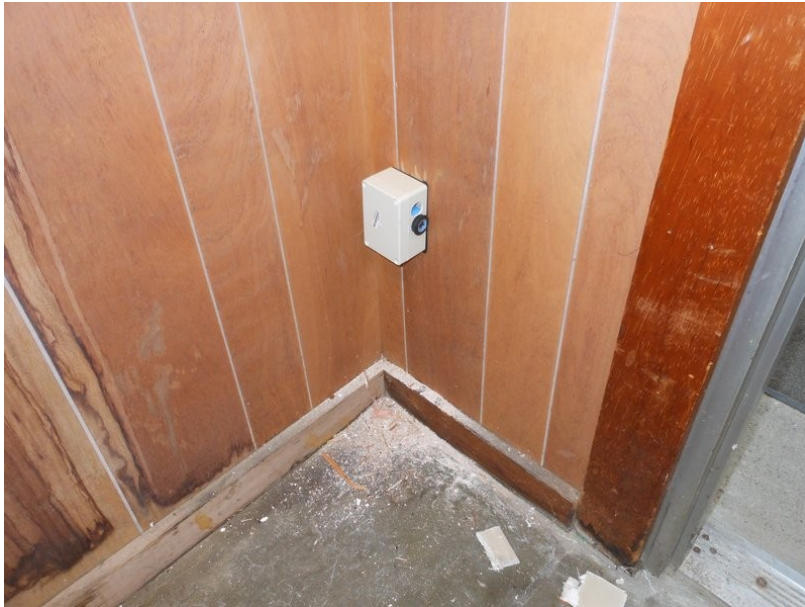
Box installed on the wall. This is a temporary box I used for testing purposes. The additional hole at the top is an error, but allows viewing the LED (though this sensor does not change its LED colour, it's always green).
